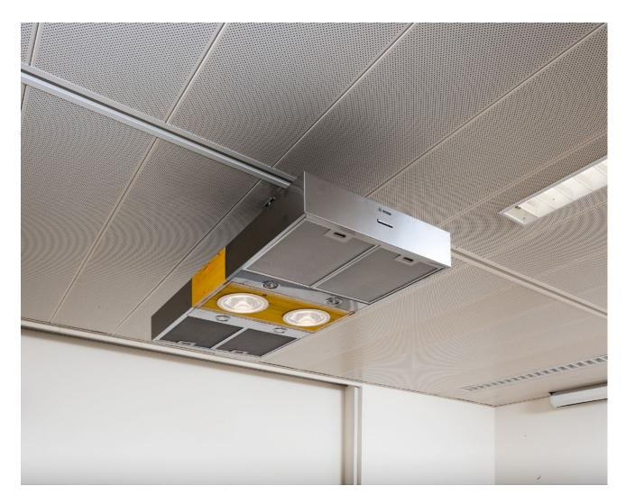
The air recirculation element consists of two standard cubic air recirculators connected together by a central box. The height of the box can be coordinated with the recirculators. Depending on the usage context, up and/or down lights can be integrated into the central element. The system is suspended by steel cables via the anchor points on the recirculators.
